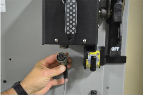
**Insert the 7 pin female straight connector into the corresponding male connector on the isoRAC® Operator. Twist the collar  $\frac{1}{4}$  of a turn to ensure positive connection. \*Note: The plugs have alignment tabs to assist with connection.**
