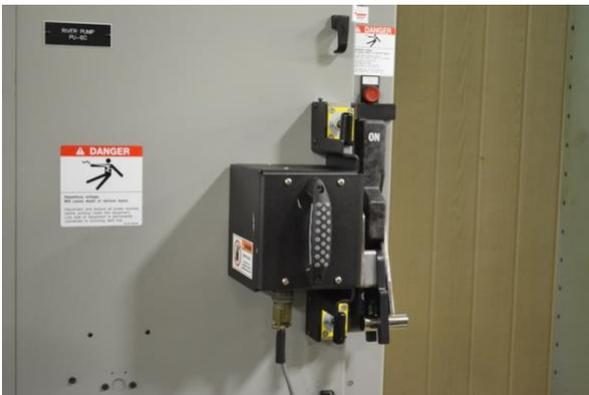
Verify the current position of the equipment Racking Handle, and be sure that you are going to Rack to the opposite position.
