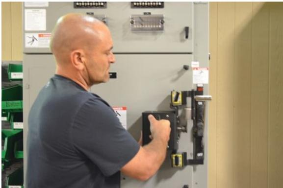
**Install the isoRAC® Operator on to the front of the equipment as shown. Be sure that the top and bottom alignment tabs are aligned with the equipment racking handle housing, and that the isoRAC® Operator arm is properly aligned with the equipment racking handle.**
