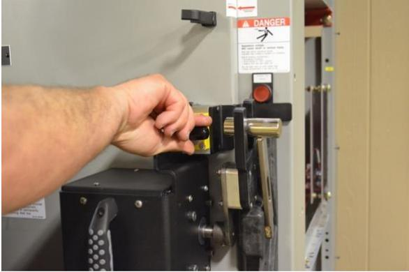
**Once the isoRAC® Operator is installed, push in and rotate the magnet handles to the “ON” position. Do this on BOTH magnets. This will hold the isoRAC® Operator in place.**
